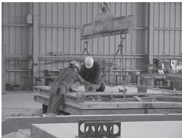
FIGURE 9.2 Precast concrete fabrication. (Photo provided by Walters and Wolf, Inc.)
