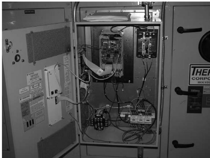
**FIGURE 40.6** Variable frequency drive (VFD). (Photo by author, courtesy of Hathaway Dinwiddie Construction Company and The California Institute of Technology.)
