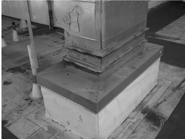
**FIGURE 40.9** Duct flashing at roof. (Photo by author, courtesy of The University of Southern California.)
