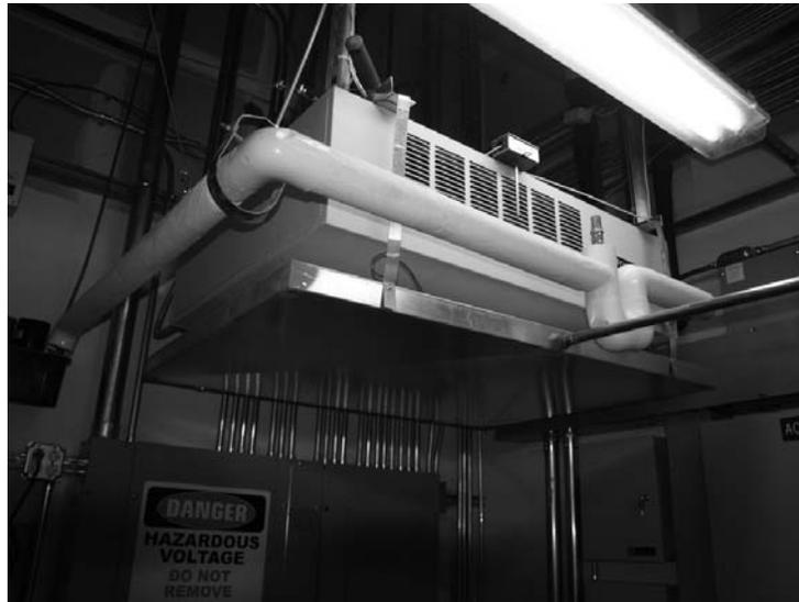
**FIGURE 40.10** Secondary drain pan. (Photo by author, courtesy of Hathaway Dinwiddie Construction Company and The University of Southern California.)
