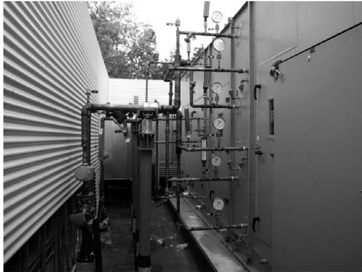
**FIGURE 40.2** Hydronic piping at an air handling unit (AHU). (Photo by author, courtesy of Hathaway Dinwiddie Construction Company and California State University Northridge.)
